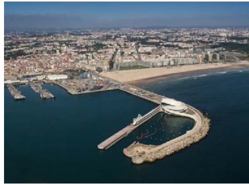
THE SITE AFTER THE INTERVENTION
