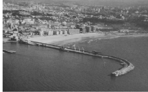
THE SITE BEFORE THE INTERVENTION
