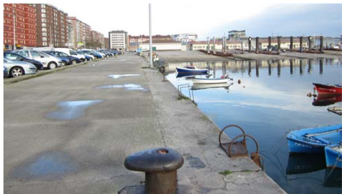
2.012 A.D. -Before the intervention-
