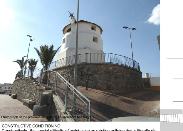
Constructively, the special difficulty of maintaining an existing building that is literally placed above our proposal arose . We had to make an excavation by bataches to build a concrete ring six meters around the base of the mill.
