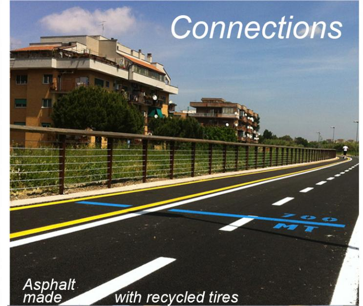
Asphalt made with recycled tires
