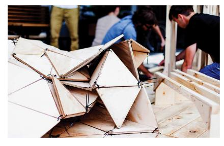
After 5 days of work two parklets were created. Each of them has approximately 11 sq.m (1.9x5.8m and 0.6m height). The floor consists of twelve metal frames fixed together and covered with the panels made of wooden planks. Over it the bicycle parking facilities were set up and the construction of the wooden triangle pieces formed the benches.
