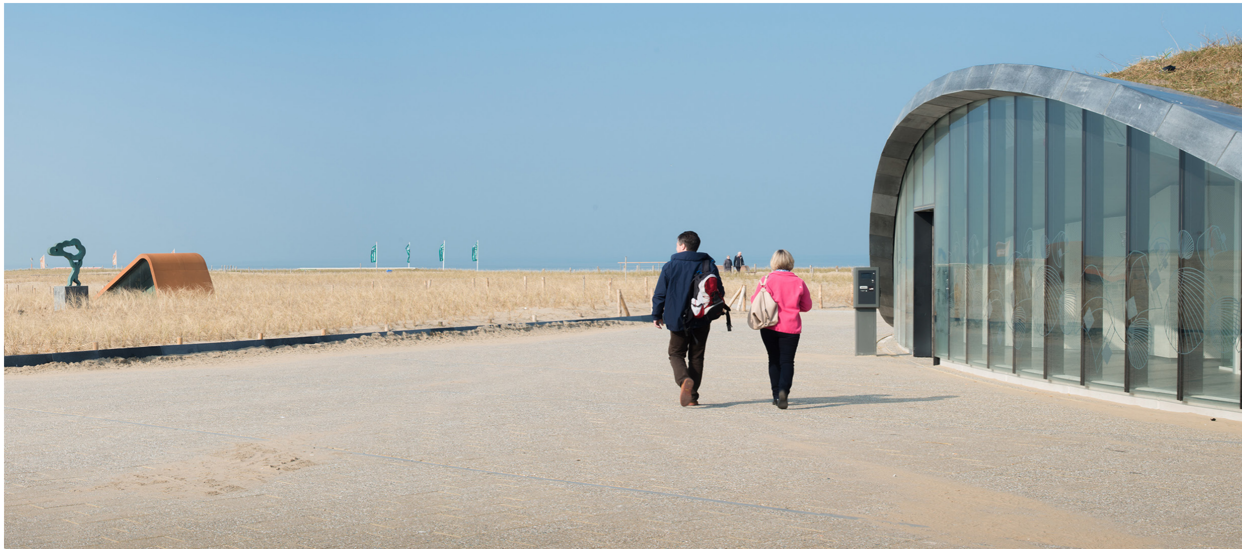
Access parking garage located at beach connection
