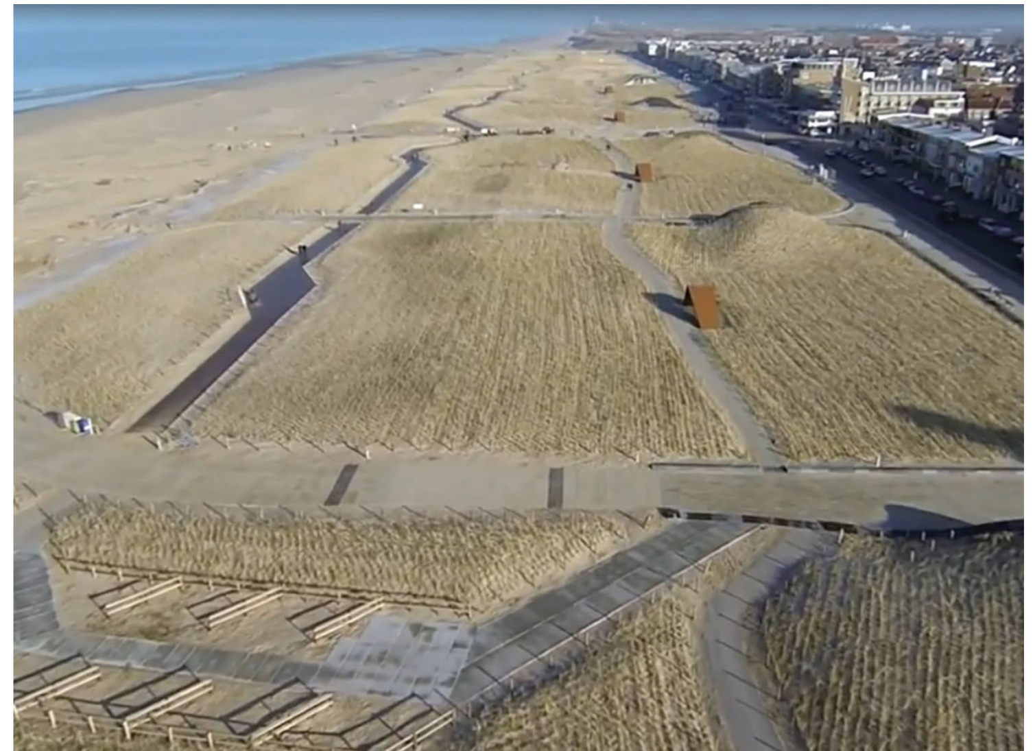
Aerial view after realisation of the coastal defense project
