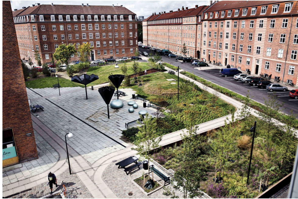
Taasinge Square combines the technical requirements of a climate-adapted urban space with the neighbourhood's desire for a green oasis and a local meeting place.
