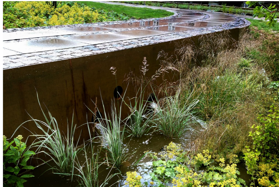
July 2015: Copenhagen's first climate-adapted urban space got its first massive downpour - and passed the test. Here the rain water is led to the "rainforest" where the plants thrive in lots of water.
