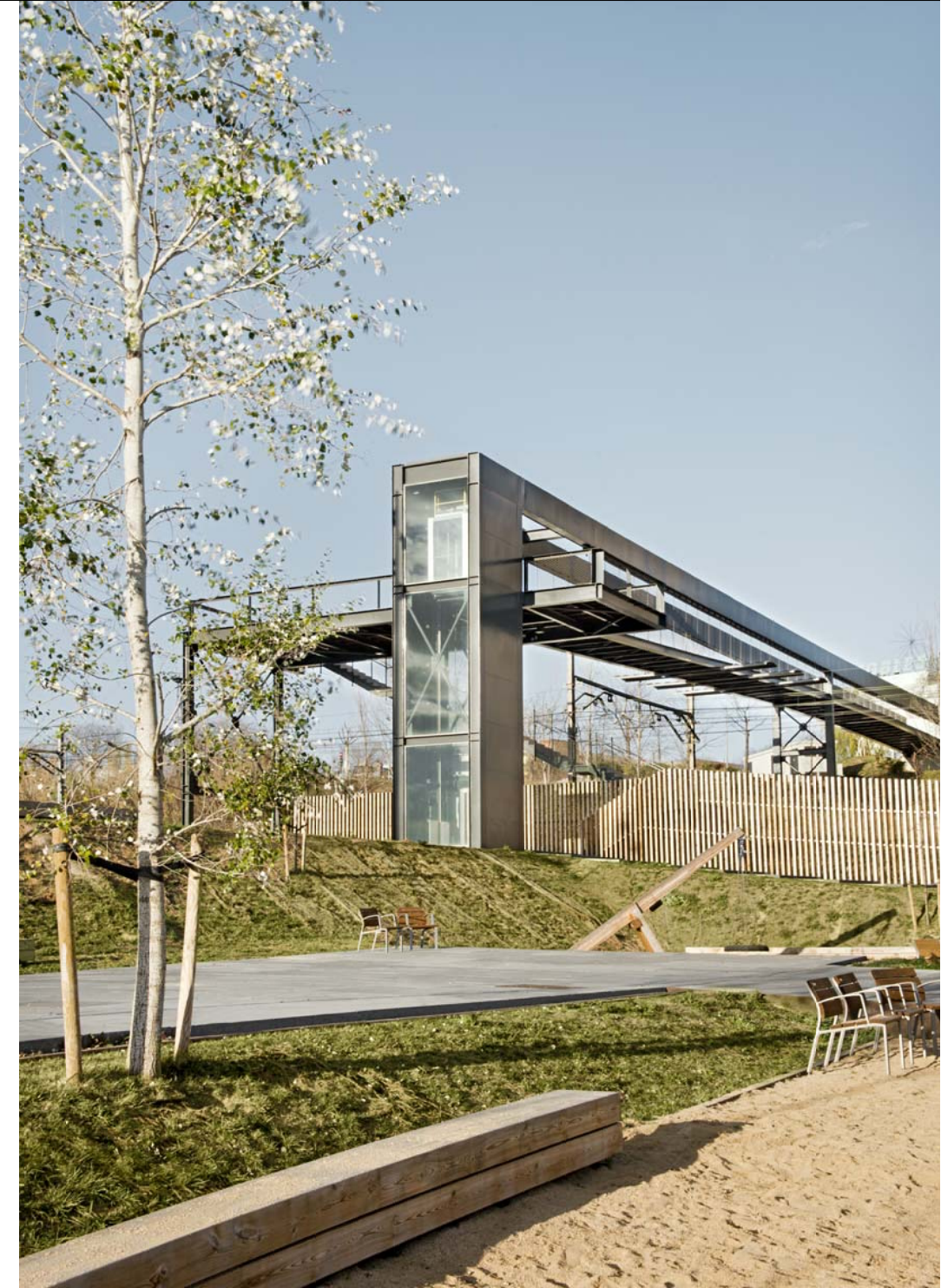
Riu Sec square and Farigola footbridge
