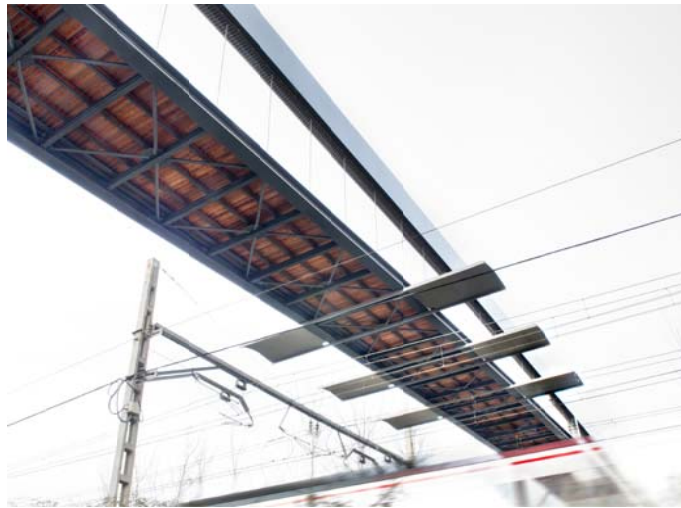
footbridge bottom view
