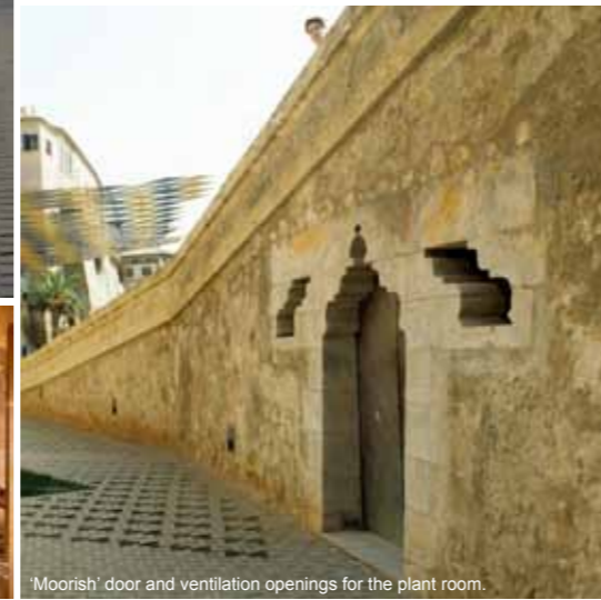
'Moorish' door and ventilation openings for the plant room.
