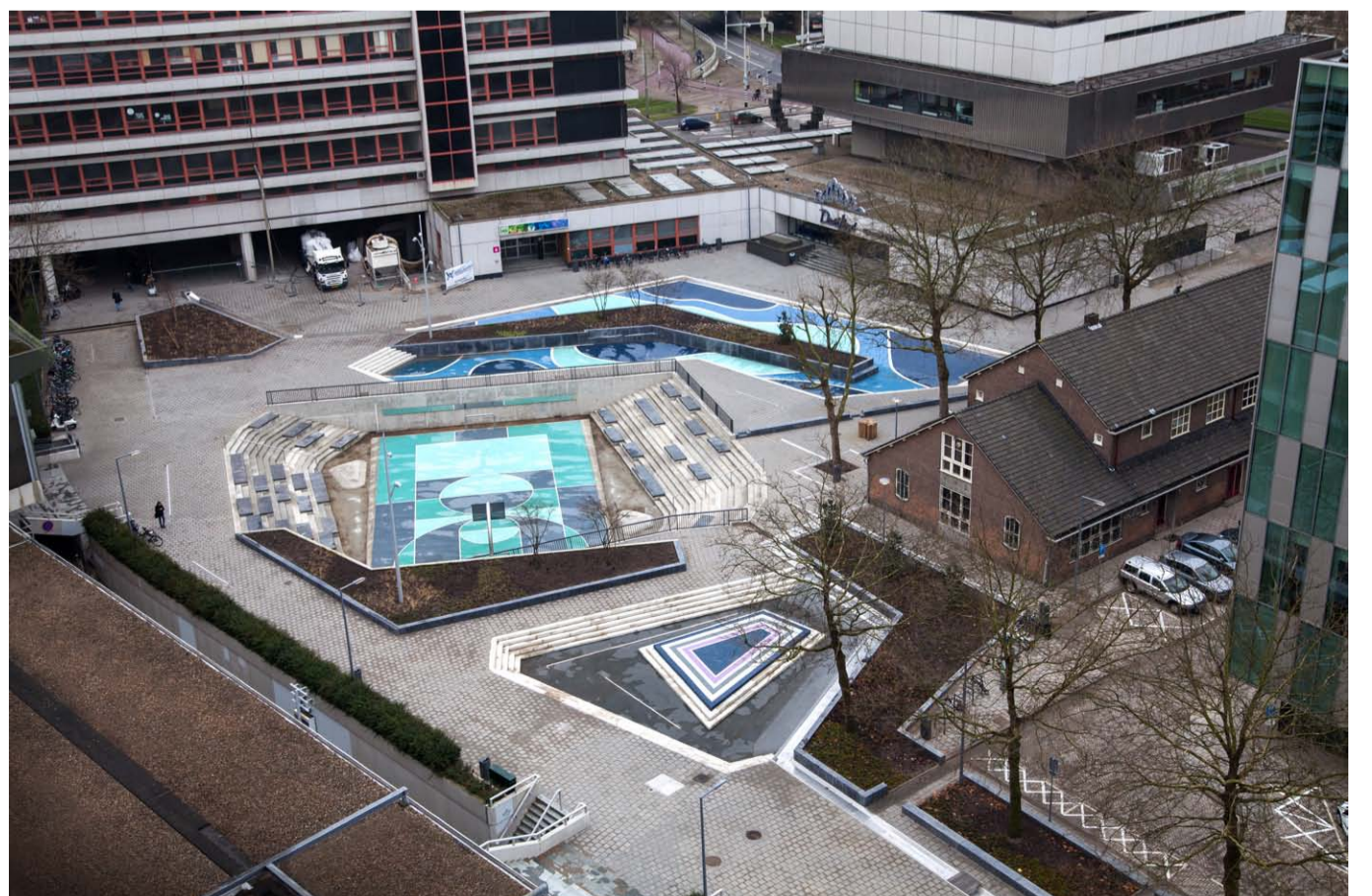
overview of the water square and its basins
