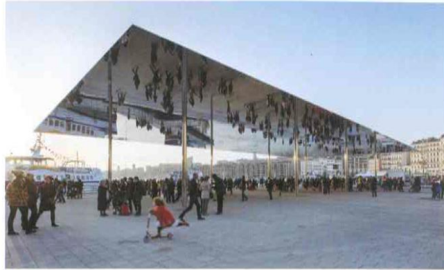
The events pavilion of the Old Port in Marseille is a canopy of highly reflective stainless steel. Its mirrored surface reflects the surroundings and tapers towards the edges, minimising its profile and reducing the structure's visual impact.
