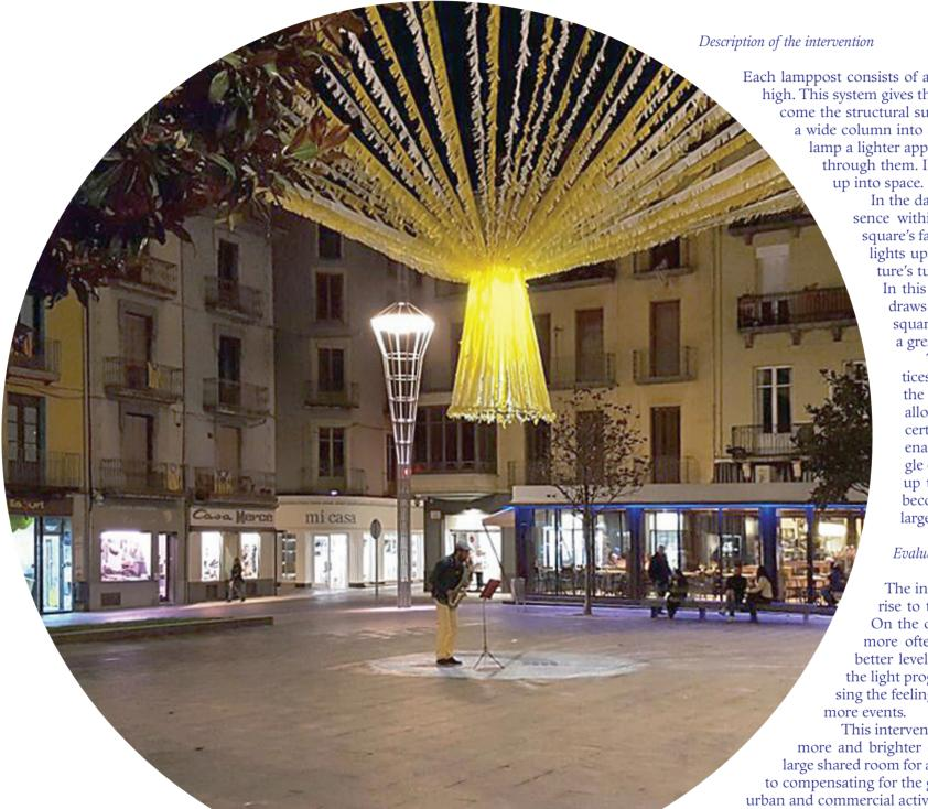
Each lamppost consists of a framed tube structure measuring 11m high. This system gives the column enough rigidness so as to become the structural support for the overhead cables. Dividing a wide column into a series of smaller tubes gives the street lamp a lighter appearance due to the fact that one can see through them. In a way they are like a line being drawn
