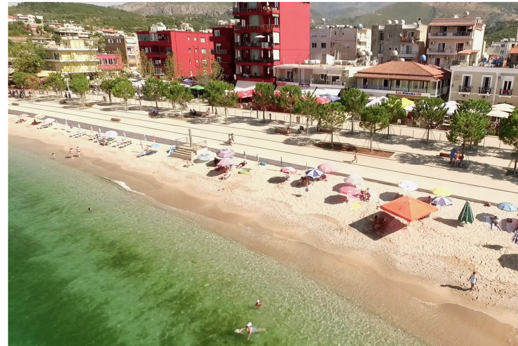
Using local sand, the platforms are made of washed concrete and appear as if the beach had been solidified.
