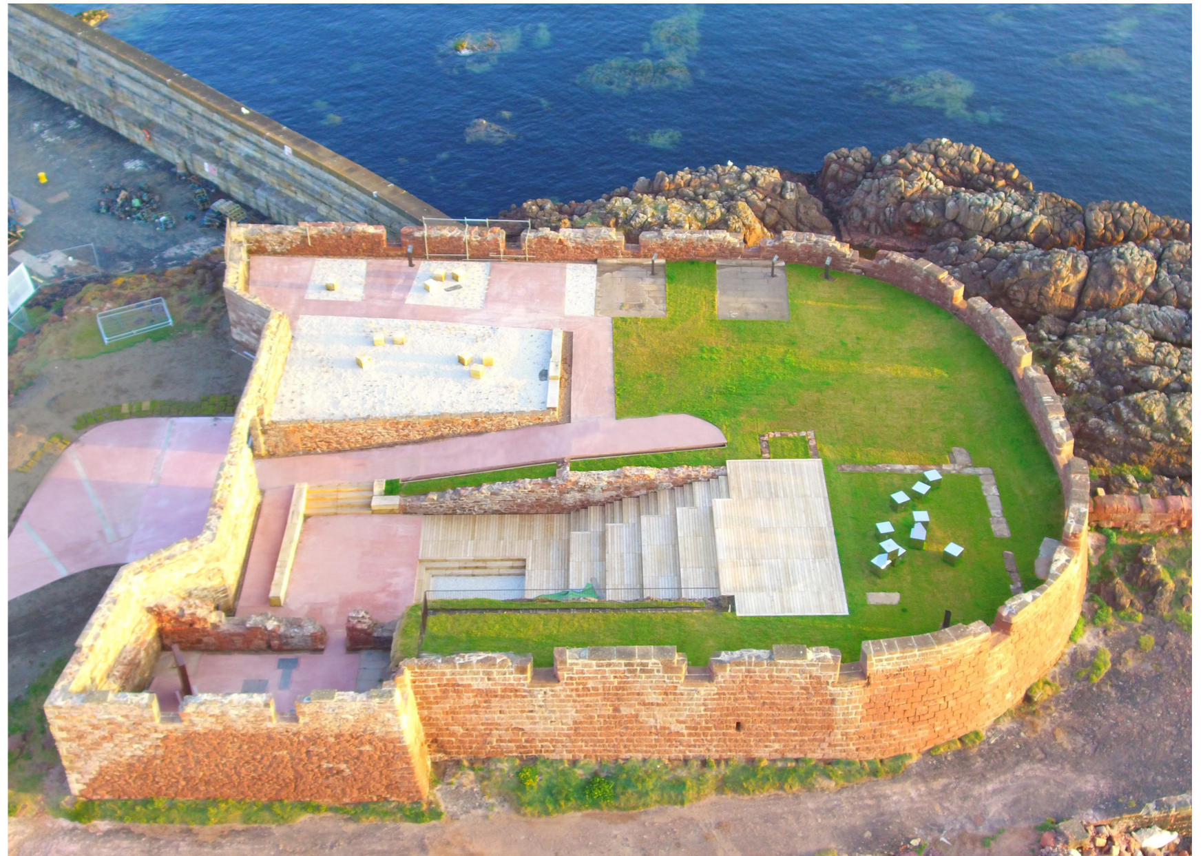
Aerial photo of completed battery project. Credit: Alistair Clark
