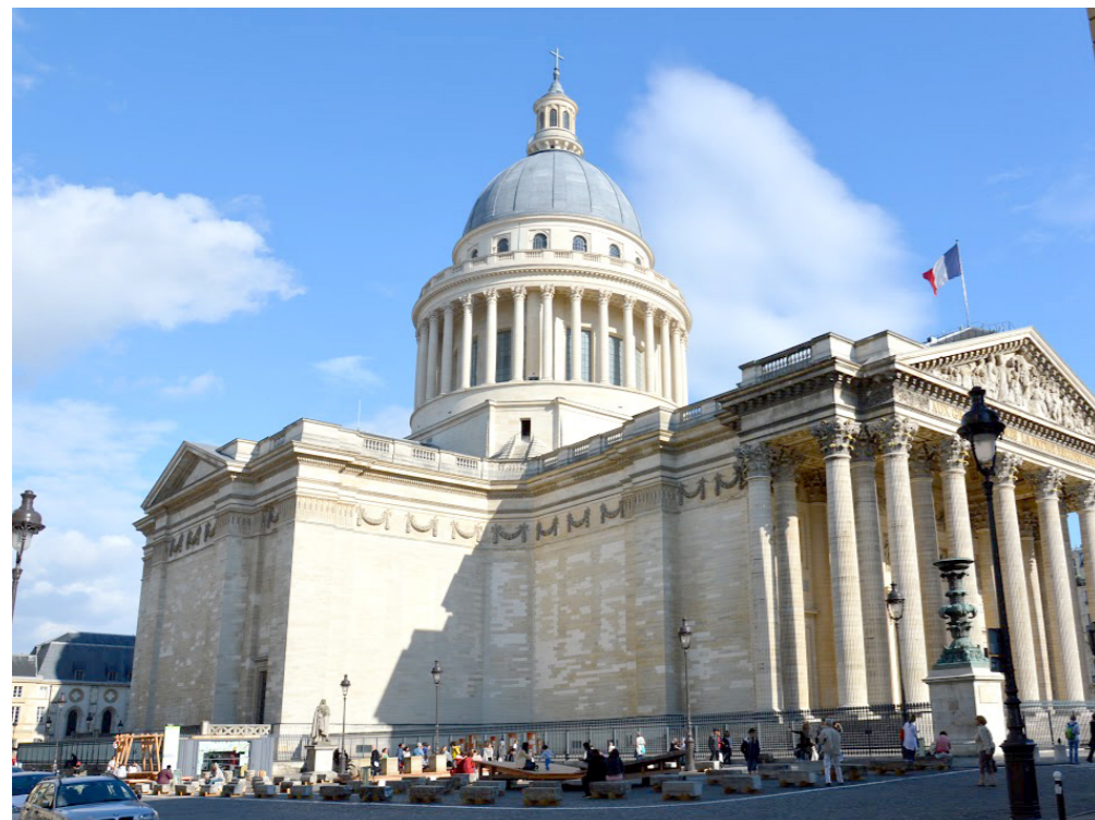
Last day of the two-weeks long construction workshop (july 2017)
