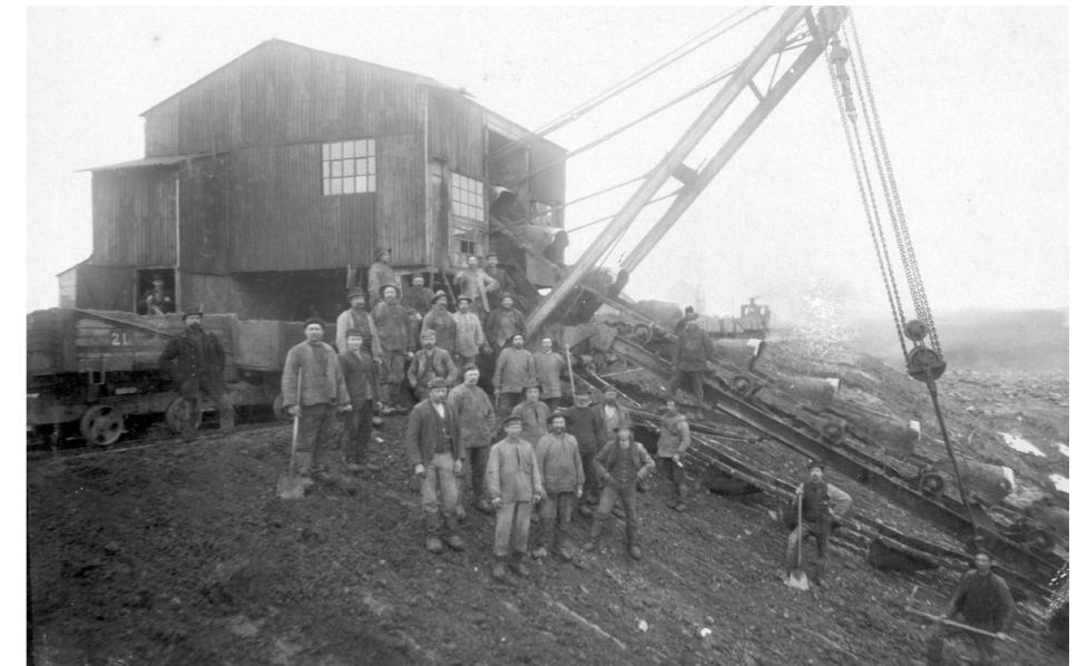
The clay quarry for the brick production from 1850. This is the area where the social housing area was later built.
