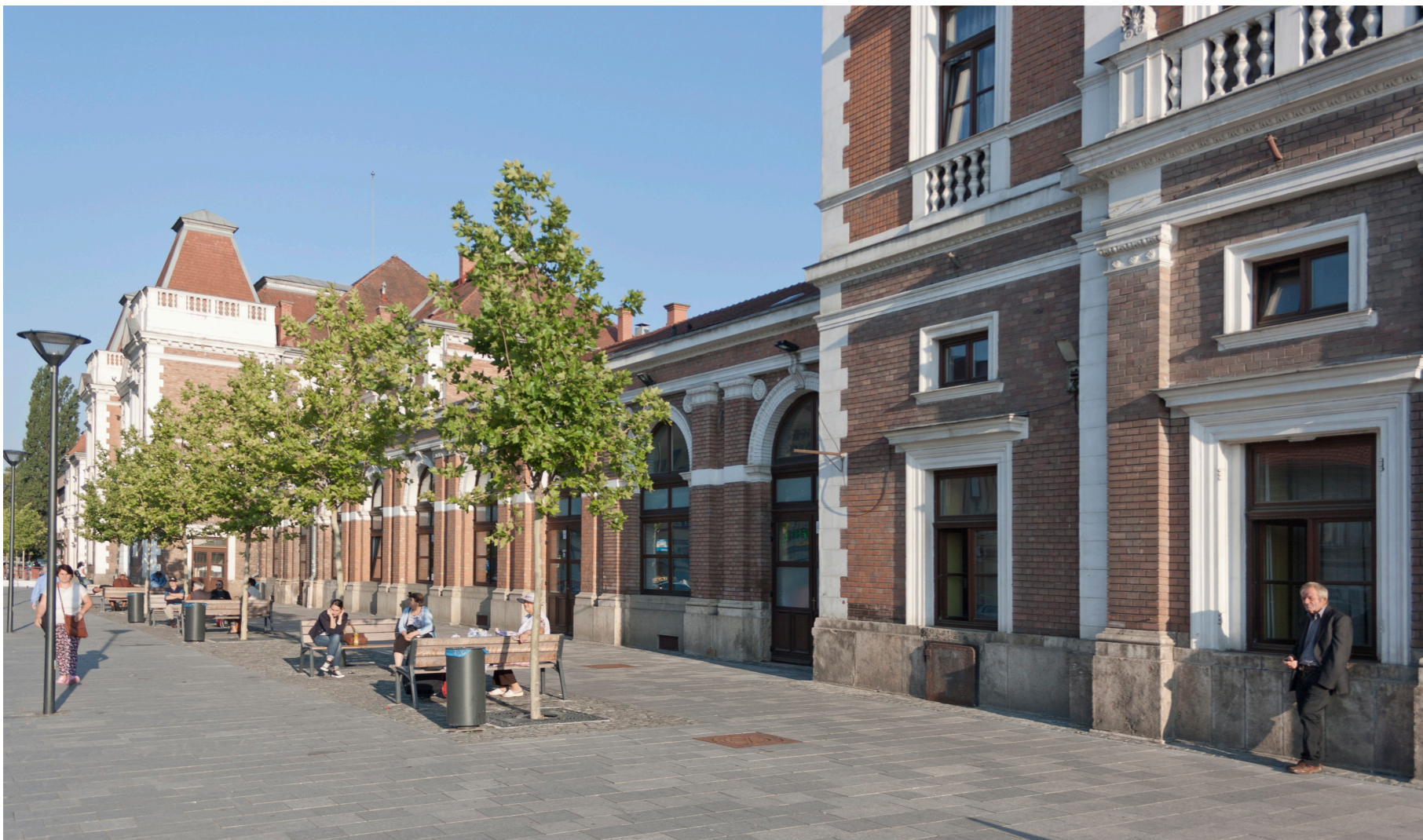
The Train Station's Square after refurbishment
