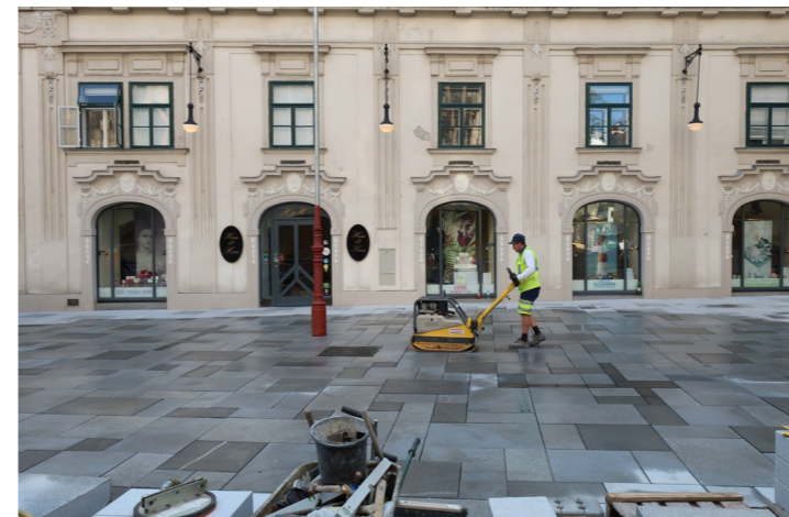
Large format plates | Construction site | August 2017
