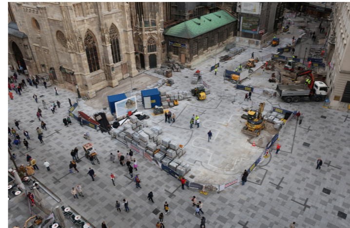
View from above | Construction site | September 2017
