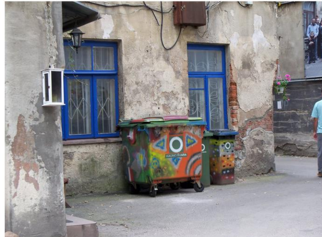
3. The Courtyard Gallery area before the intervention.
