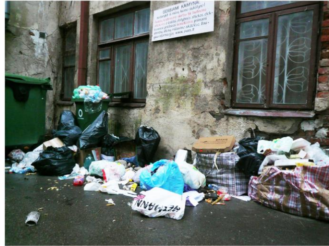
2. The Courtyard Gallery area before the intervention.
