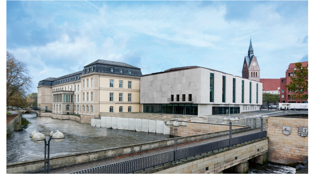
Heritage listing – a true new build was realized behind the rejuvenated, heritage-listed façade.
