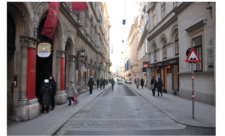
Before the intervention
