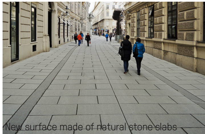
Levelled redesign of the new street surface
