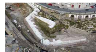
Bastion BEFORE the intervention
