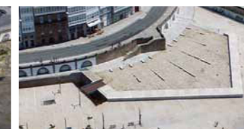
Bastion AFTER the intervention
