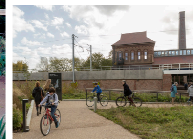
The main route is of generous width to allow shared cycle and pedestrian use
