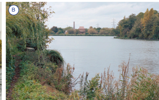
A vantage point at the edge of Reservoir no. 1 looking towards the Marine Engine House
