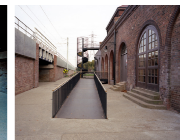
Exposed aggregate concrete and weathered steel plate of the entrance steps and ramp
