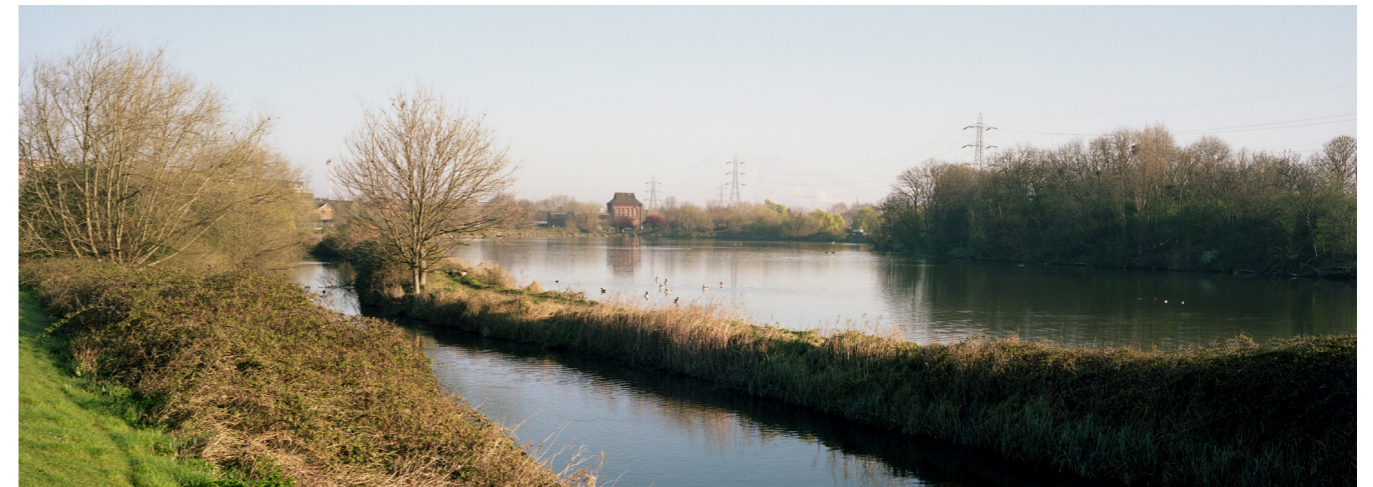
A view north across the Coppermill Stream and Victorian Reservoir 1 to the Engine House
