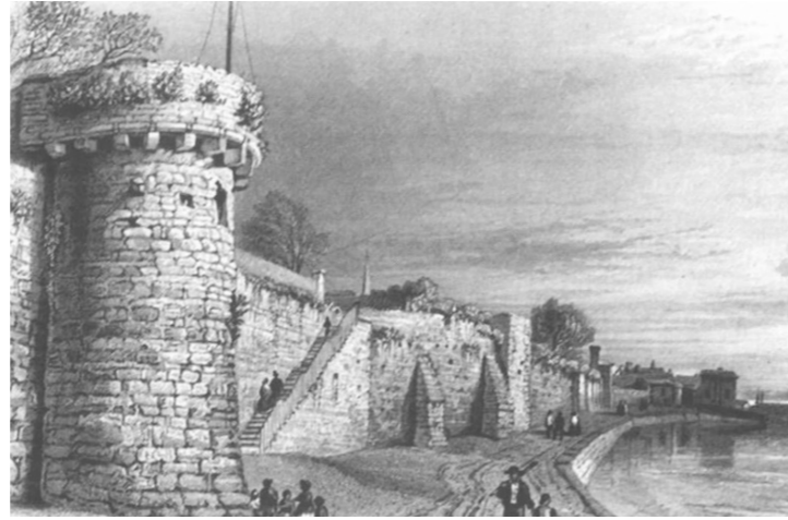
view south along town wall 1780
