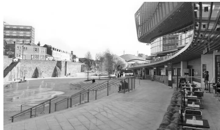
View south along town wall 2017
