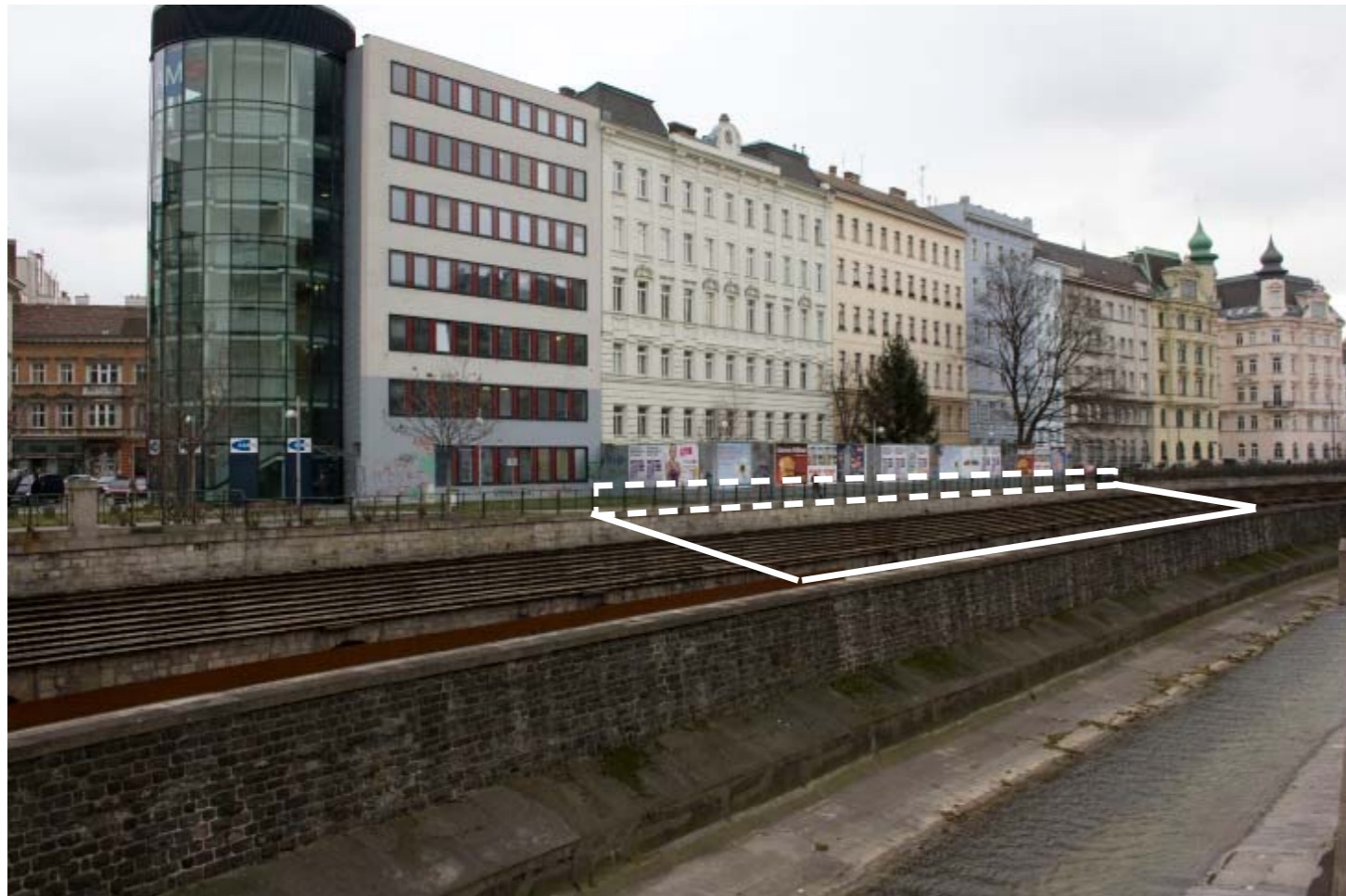
Before the intervention: The site of the Vienna Valley Terrace consisted of the subway tracks on one hand and a left-over space hidden behind billboards on the other side.
