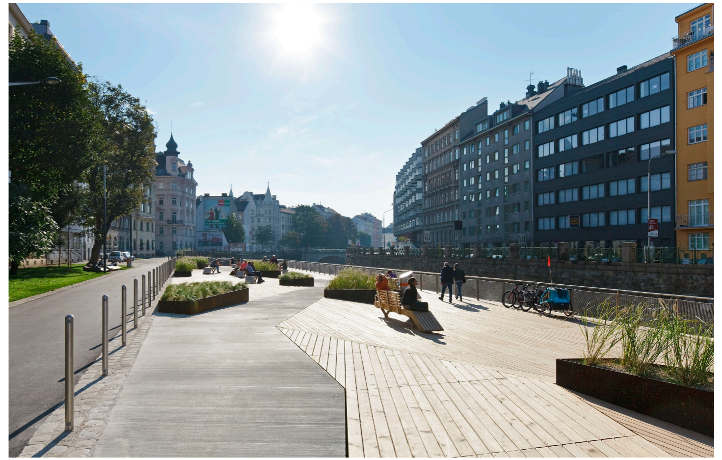
After the intervention: The Vienna Valley Terrace creates new, free, non-commercial public space and integrates footpaths and bicycle paths with the metro line.
