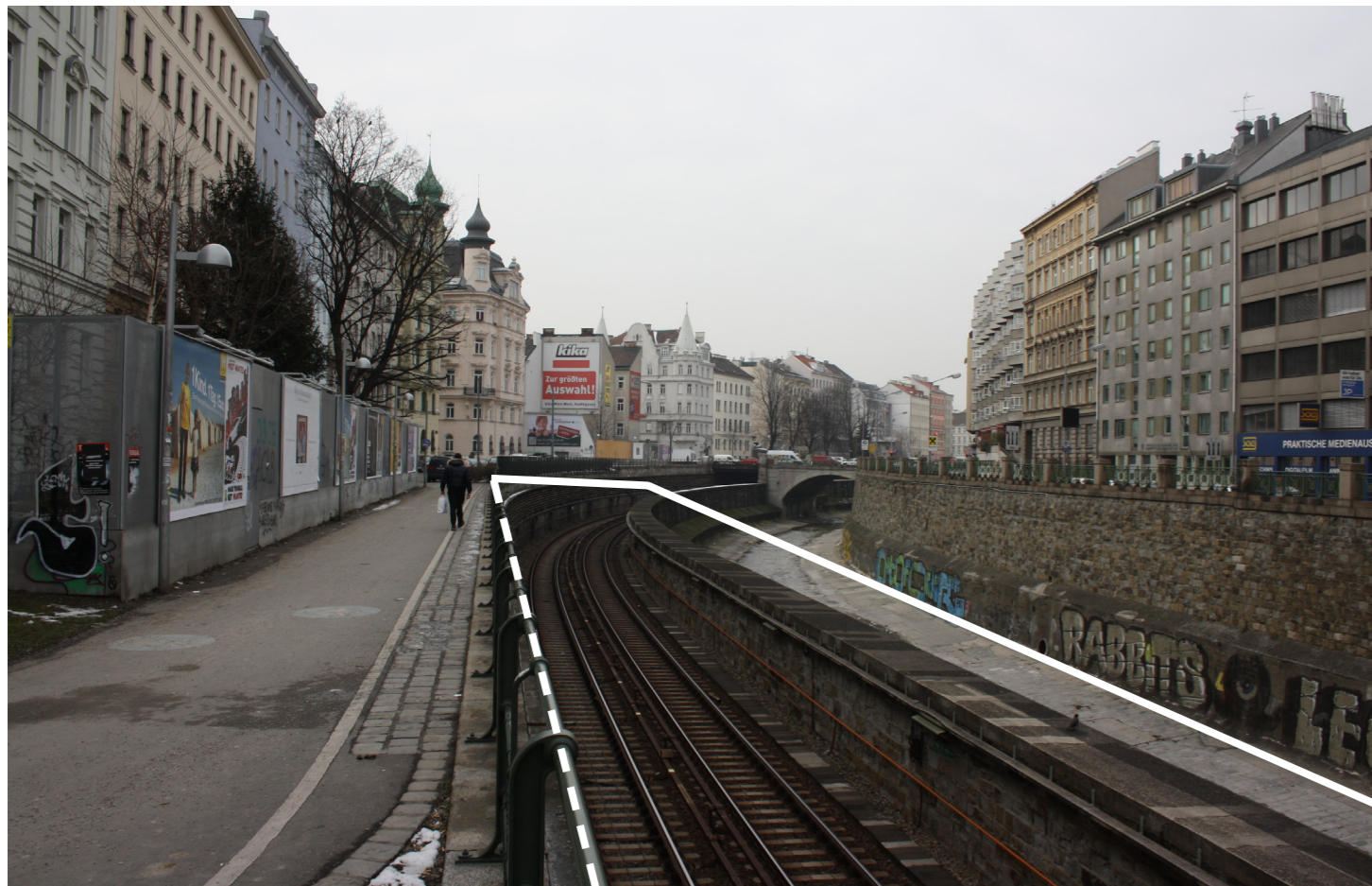
Before the intervention: Cramped in between the tracks and the billboards was a narrow footpath combined with a bicycle lane - a dangerous situation with a blind corner that frequently led to collisions.
