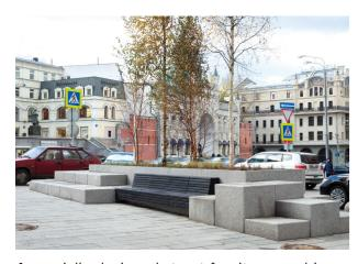
A specially-designed street furniture combines planters and sitting places. This is a perfect solution to be used on a street, where planting trees is impossible due to a large amount of underground communications. The size and construction of the planterns are preventing the ground from freezing, therefore the trees can survive the cold Russian winter and don't need to be replaced each year.
